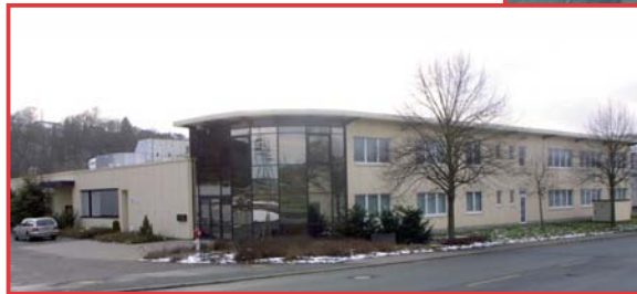
New plant in Asslar
